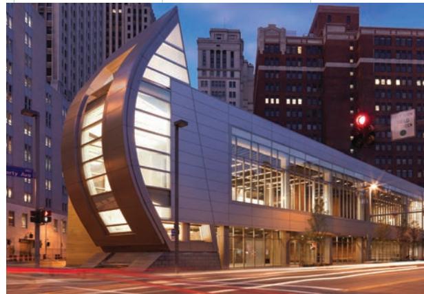
1999 – The Foundation awards a $25,000 planning grant to study a proposed African-American cultural facility in Downtown Pittsburgh. Today, and with the help of nearly $20 million in Foundation support, it is the August Wilson African American Cultural Center.
