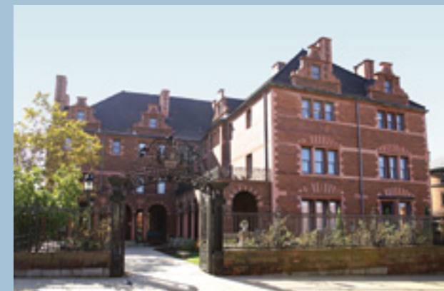
Byers Hall at Community College of Allegheny County's North Side campus
