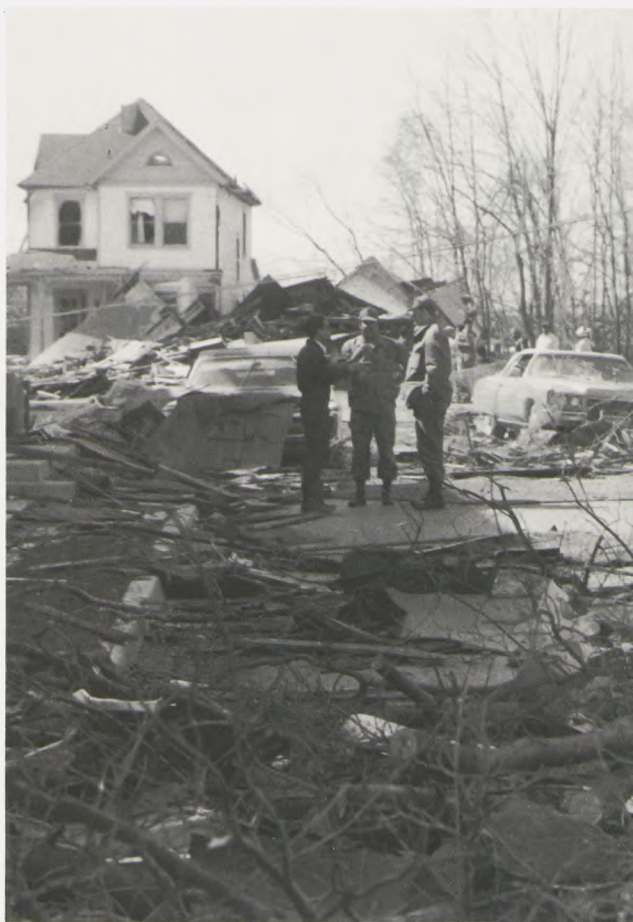
Wilberforce University: These two photographs are representative of the widespread destruction on the campus due to the tornado which, in a matter of minutes, did more than $5,000,000 damage.
