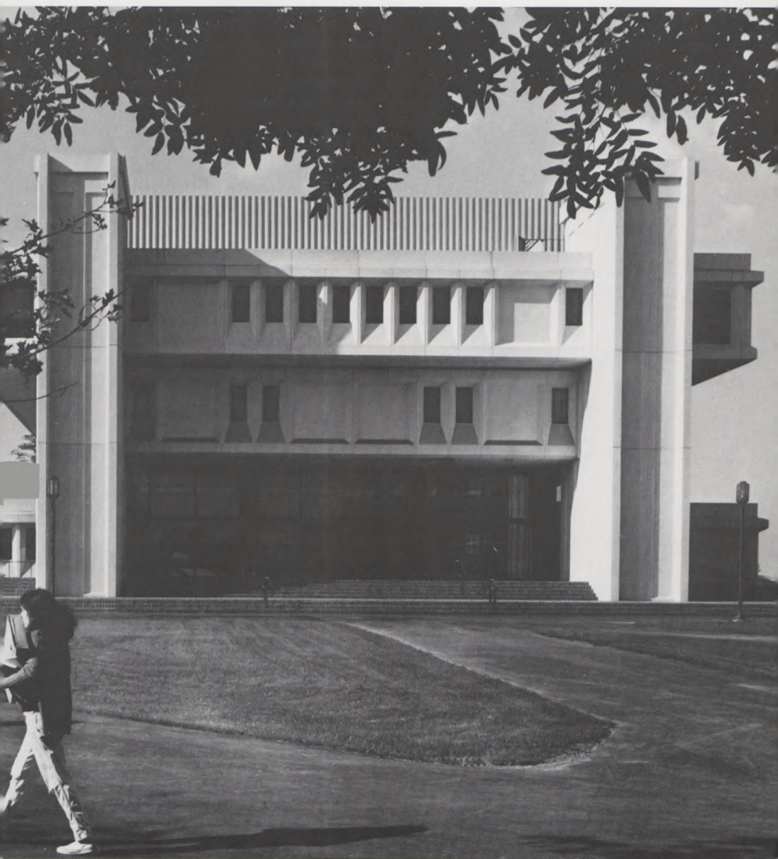
The entrance facade of the Jennie King Mellon Library, Chatham College. The Library is designed for 200,000 volumes. One-story wing at left connects the Library with a small theatre.
