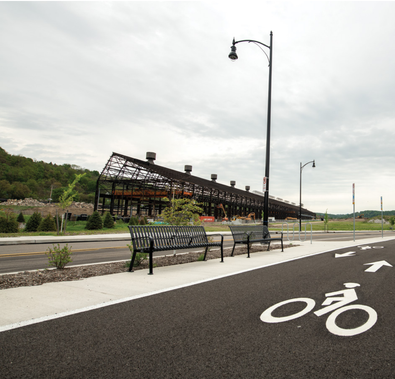
The Mill 19 building will serve as the anchor property at Hazelwood Green and as the headquarters for Carnegie Mellon University's Advanced Robotics for Manufacturing Institute and Manufacturing Futures Initiative.
