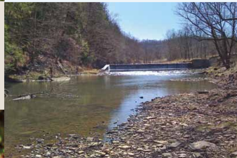
Dunkard Creek's low-head dam (before, above left) in Greene County, Pennsylvania, was built in 1910 to provide water for a natural gas compressor station. The use was abandoned in the 1950s. American Rivers has provided technical assistance and funding to the present dam owners for the dam's deconstruction and to restore the adjacent riparian border (after, above right).
