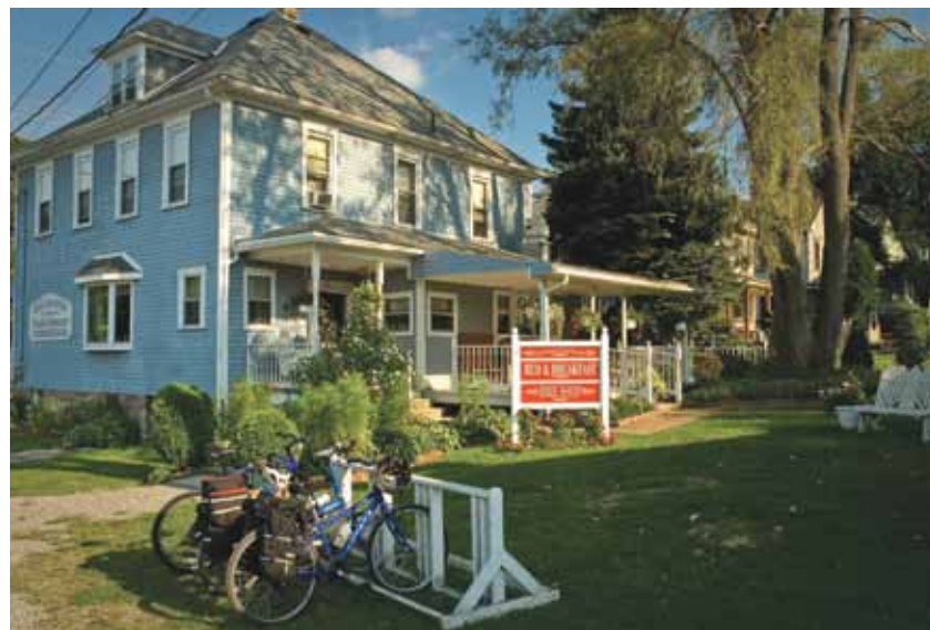
In Rockwood, adjacent to the Rockwood Trail Bed & Breakfast, The Progress Fund is making safety and signage improvements to the Great Allegheny Passage trailhead, including building a sidewalk that will provide safer travel into the town's center.
